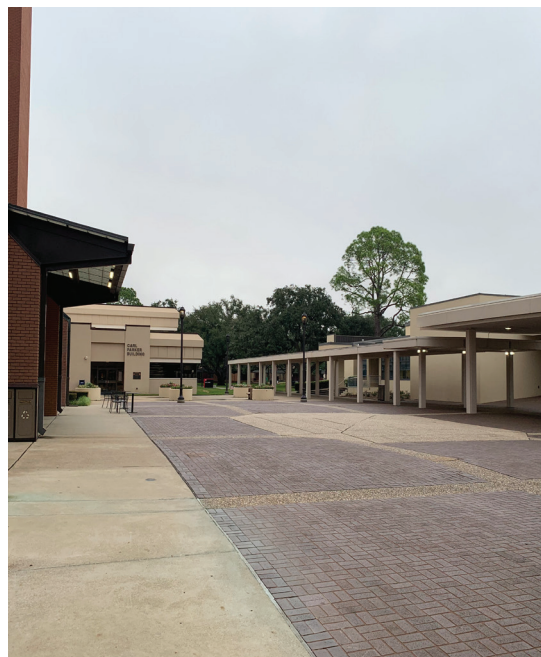
Existing East Entry Plaza
